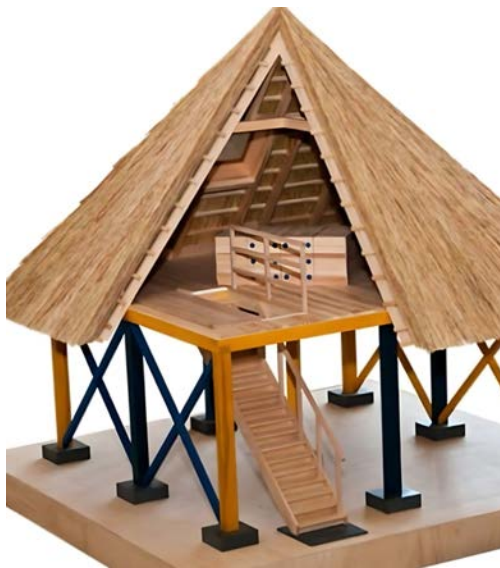
Fig. 1. Model of the Apitherapeutic Pyramid: general view of the structure with hive module, access stairs to the working platform, and support frame (visualization sample for describing the structural elements of the patented product)
